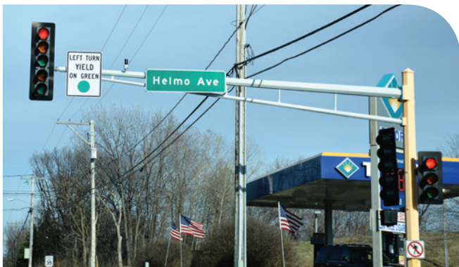
Oakdale has reduced its costs for energy consumption and maintenance by using LED technology in all signal lights.
